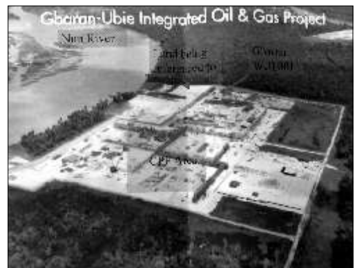
Gbarain/Ubie Integrated Oil and gas Project, in Obunagha Community
